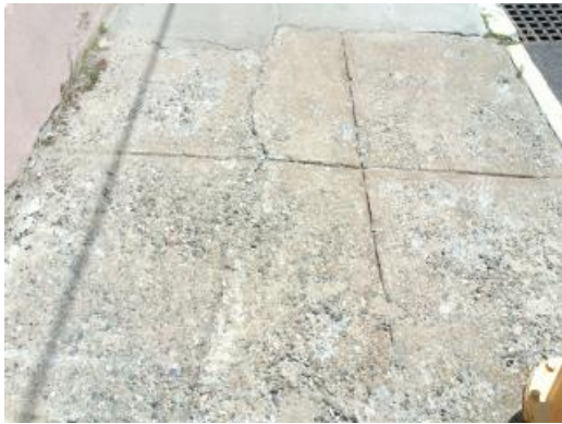
Spalled Sidewalk
