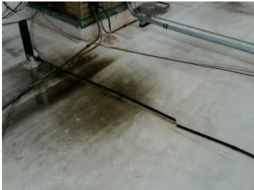
Abandoned Equipment On Roof
