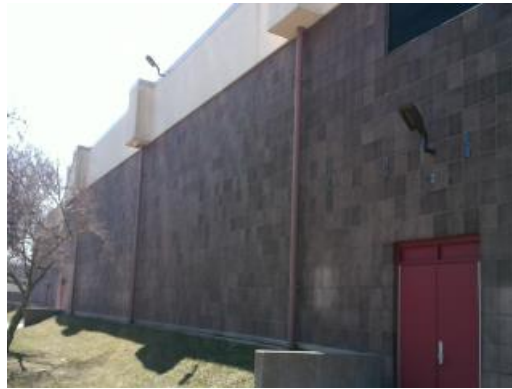
Main Building - Exterior Finishes
