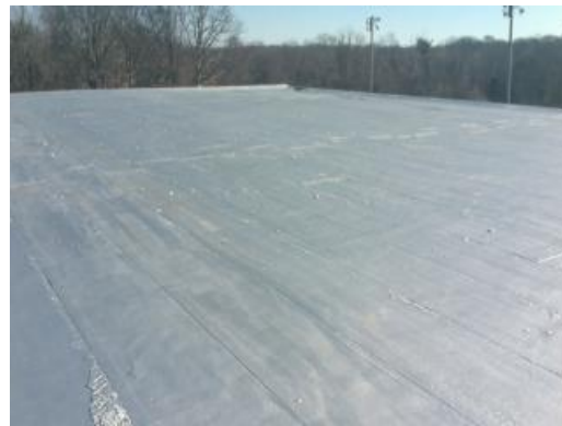
Roof General Condition
