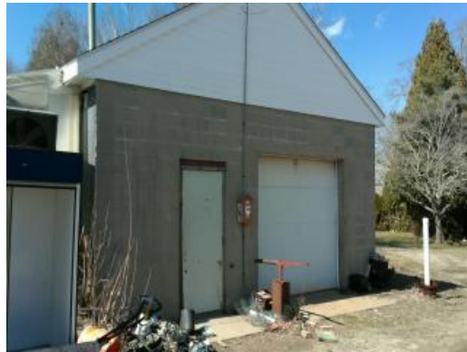
Building 03 - Exterior Finishes
