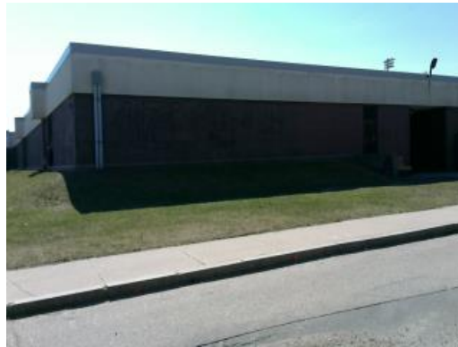
Main Building - Exterior Finishes
