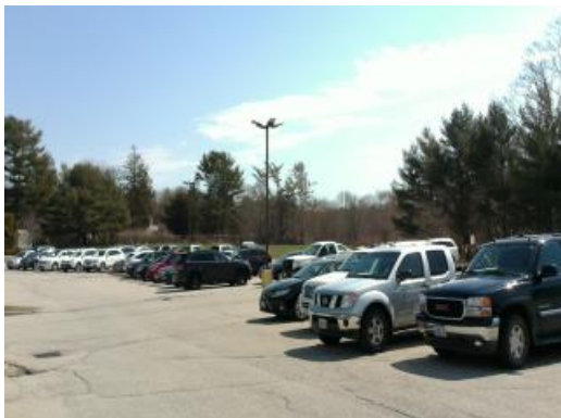
Typical Pole Lights
