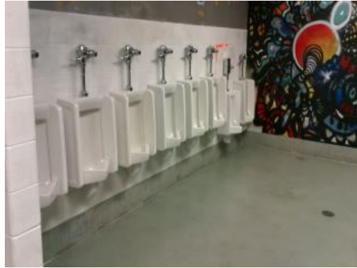
Main Building - Original Urinals
